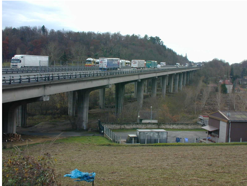
Figure 1. Bridge considered in the study.
