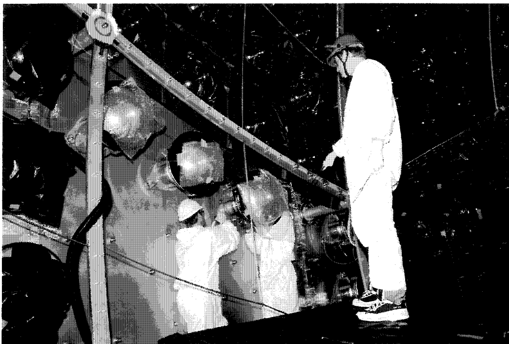
Figure 3.2: A photograph of PMT installation. The workers are, from left to right, K. McKinny (University of Alabama), the author, and J. Ritter (California Institute of Technology). Photo taken by T. Takayama (Tohoku University).
