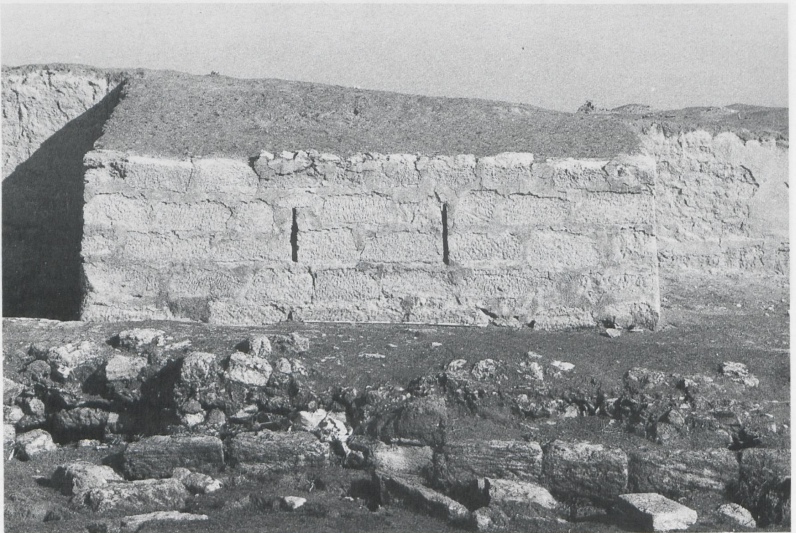
Fig. 5 - Tower 1 from the front. In the foreground, remains of the proteichisma .
