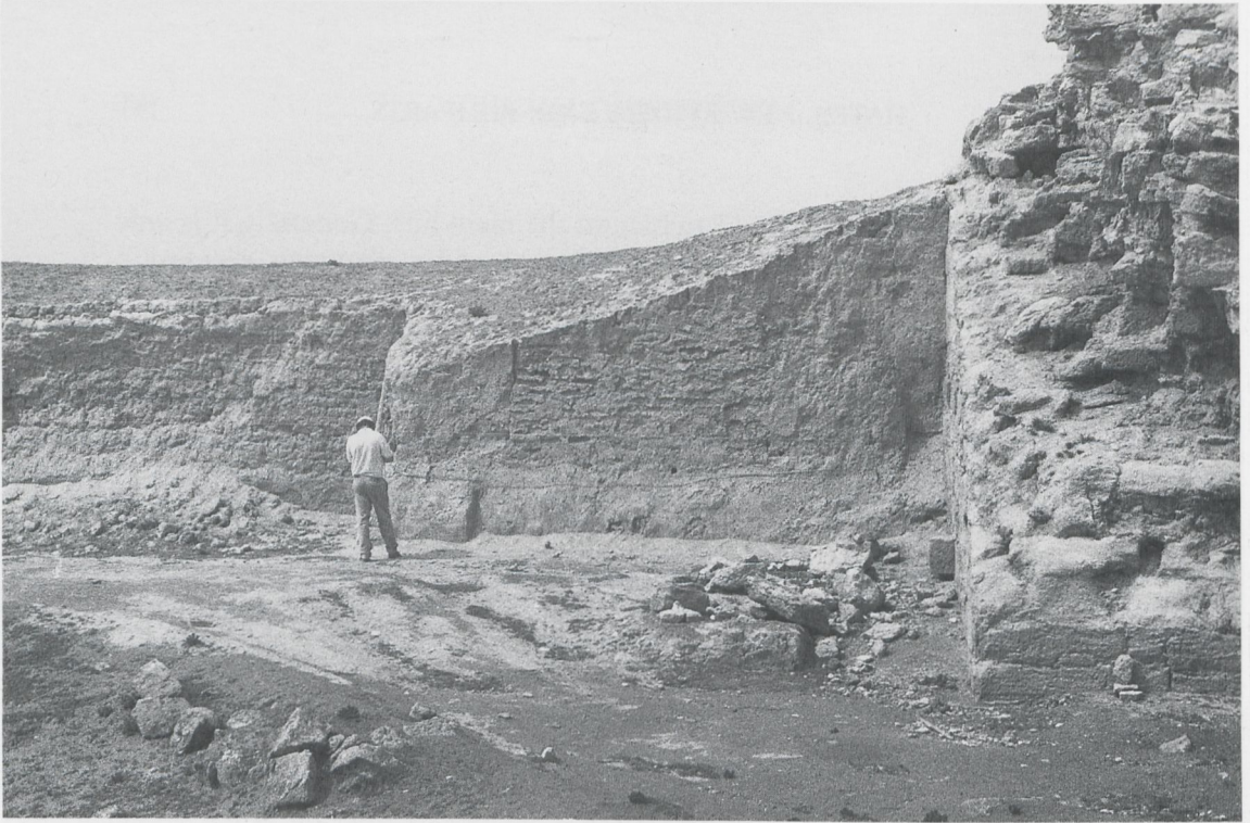
Fig. 9 - Tower 10, cut and filled with mortar-held bricks.
