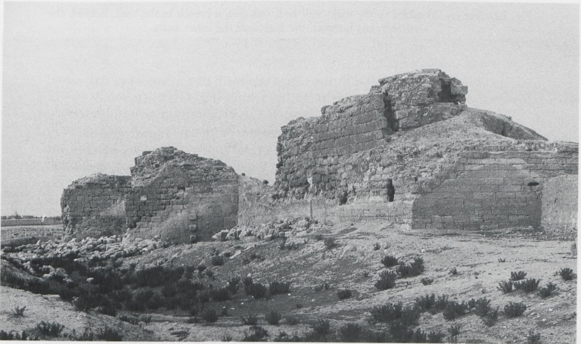
Fig. 11 - A view of the eastern front: right, an incorporated tomb, behind a late stone curtain, then batteries 11 and 8.
