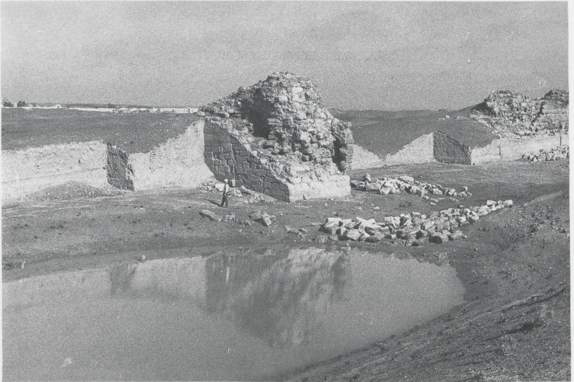
Fig. 4 - Part of the main wall: tower 10 and battery 11. The enlarged ditch is filled with rainwater.
