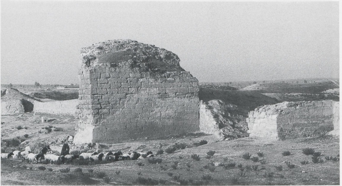
Fig. 12 - Battery 20 added to the main wall and, this side, a breach in the wall. Behind, the enclosed area between the main and the inner walls.
