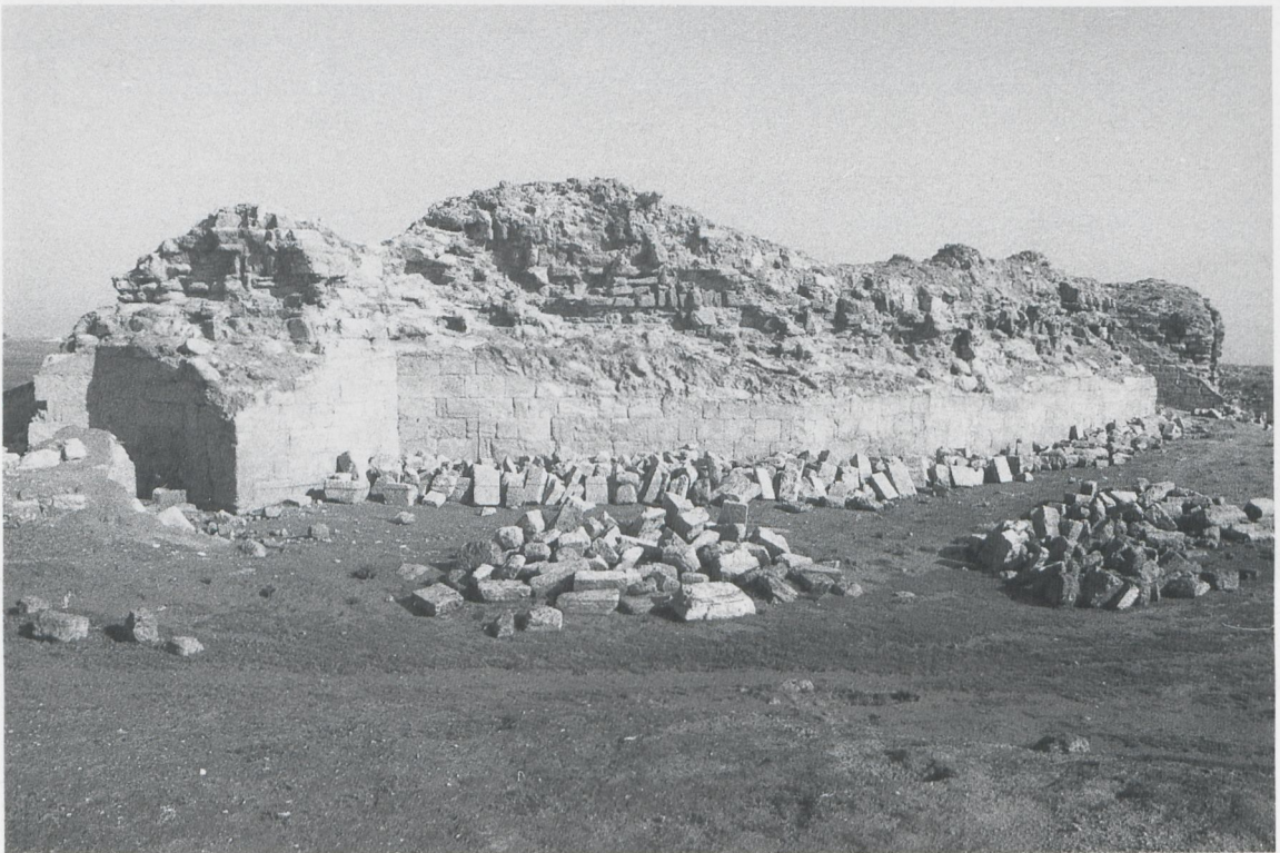
Fig. 10 - The SE corner bastion and stone curtain doubling the original mudbrick rampart (sectors 4 and 5).
