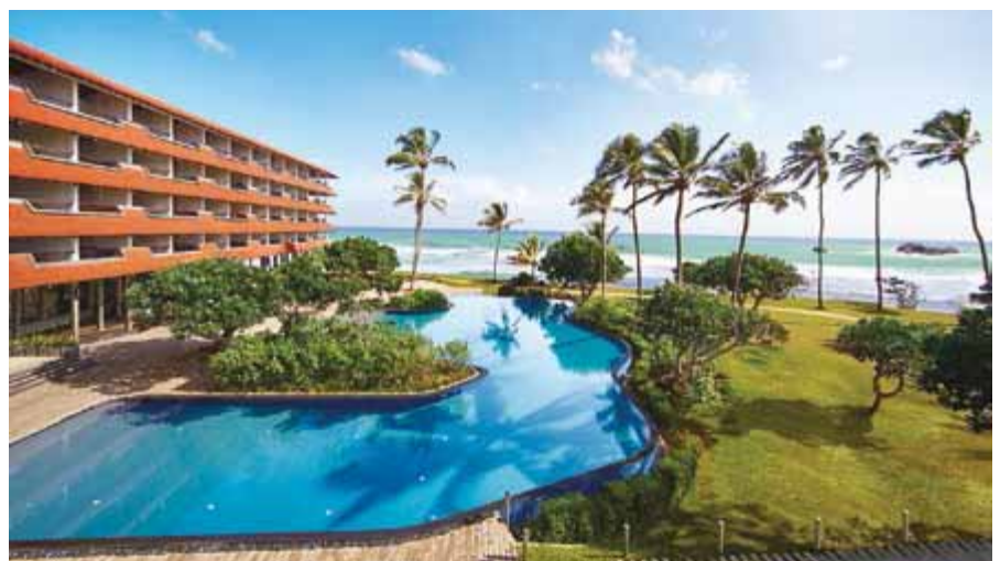
'Hikka Tranz by Cinnamon' re-opened in May 2021 following the completion of structural repairs.
