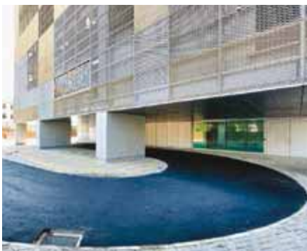
Asphalt Road at 'Cinnamon Life', together with AGC Innovate.
