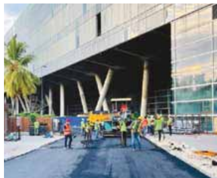
Construction of Asphalt road at 'Cinnamon Life'.
