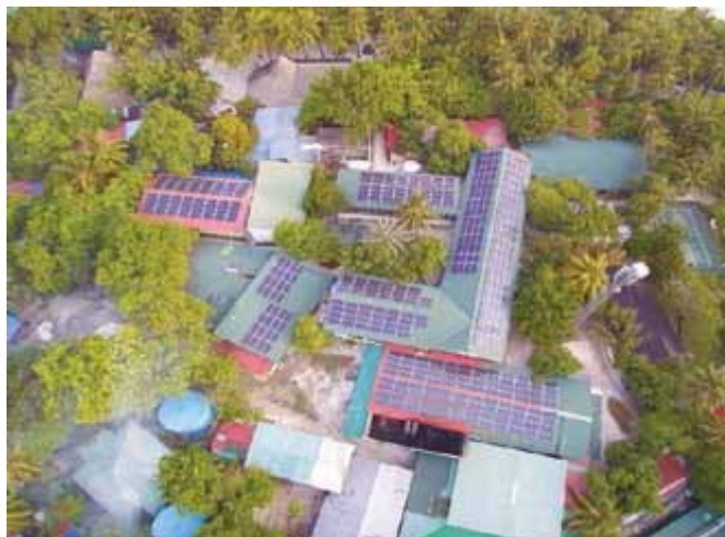
Solar panels at 'Ellaidhoo Maldives by Cinnamon'.
