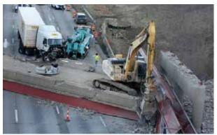
**University of Cincinnati** architecture professor Tom Bible said the pictures indicate a failure of the joints at the western joint of the span. That wouldn't have happened, he said, if the eastern end of the bridge over the median and connecting to the old Hopple Street connection hadn't been previously removed. "Judging from the pictures, it obviously slipped off its supports," he said.
