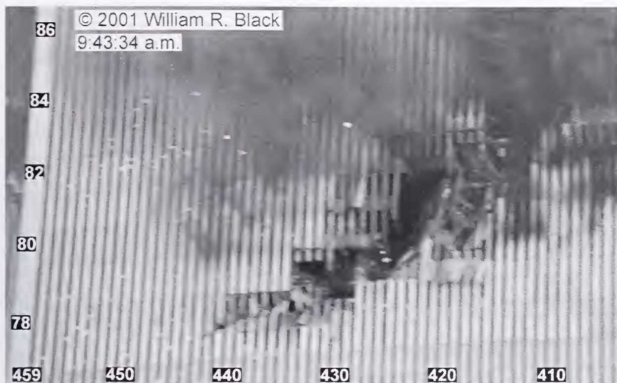
Figure 9-56. This cropped, slightly out of focus photograph of the south face of WTC 2 was shot at 9:43:34 a.m. The intensity levels have been adjusted, and column and floor numbers have been added. The flames visible to the left of the western edge of WTC 2 are on the south side of WTC 1.
