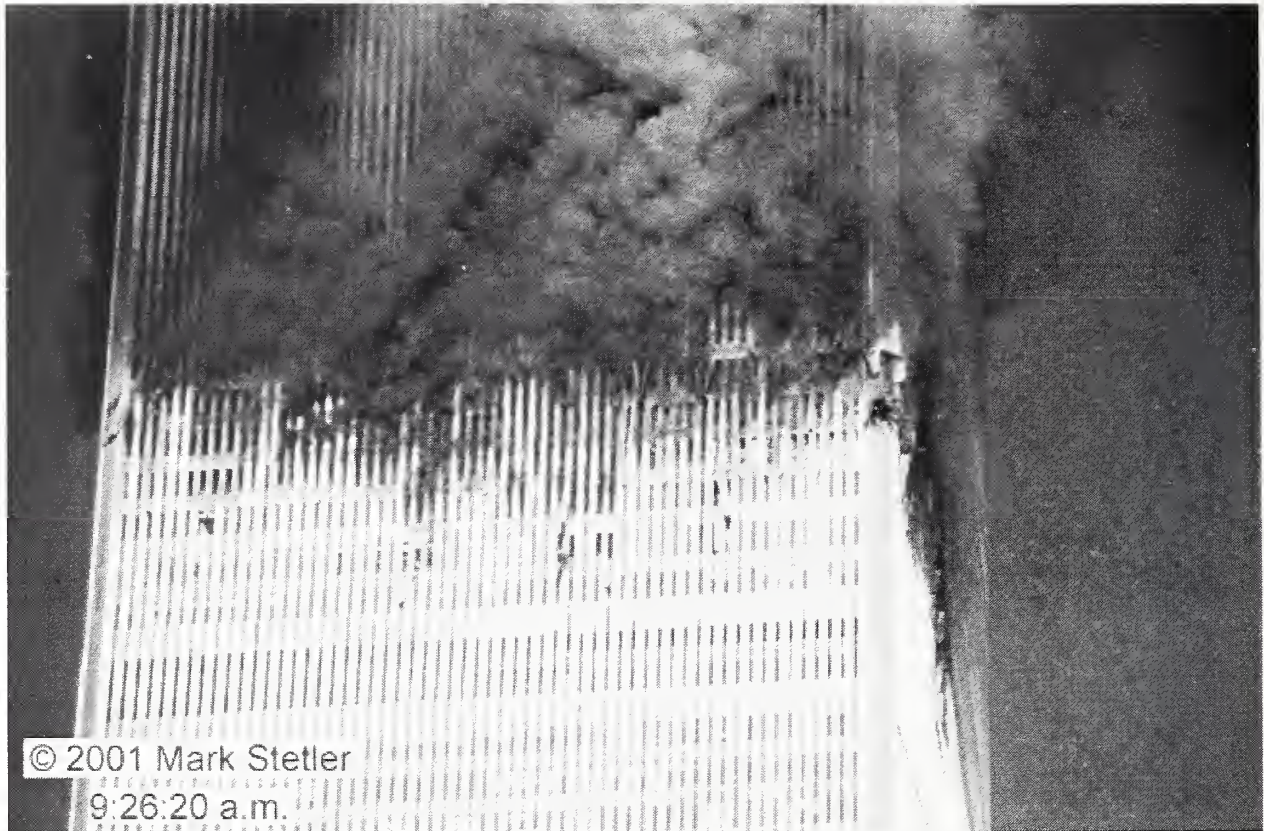
Figure 9-30. This photograph showing the east face of WTC 2 was taken at 9:26:20 a.m.
