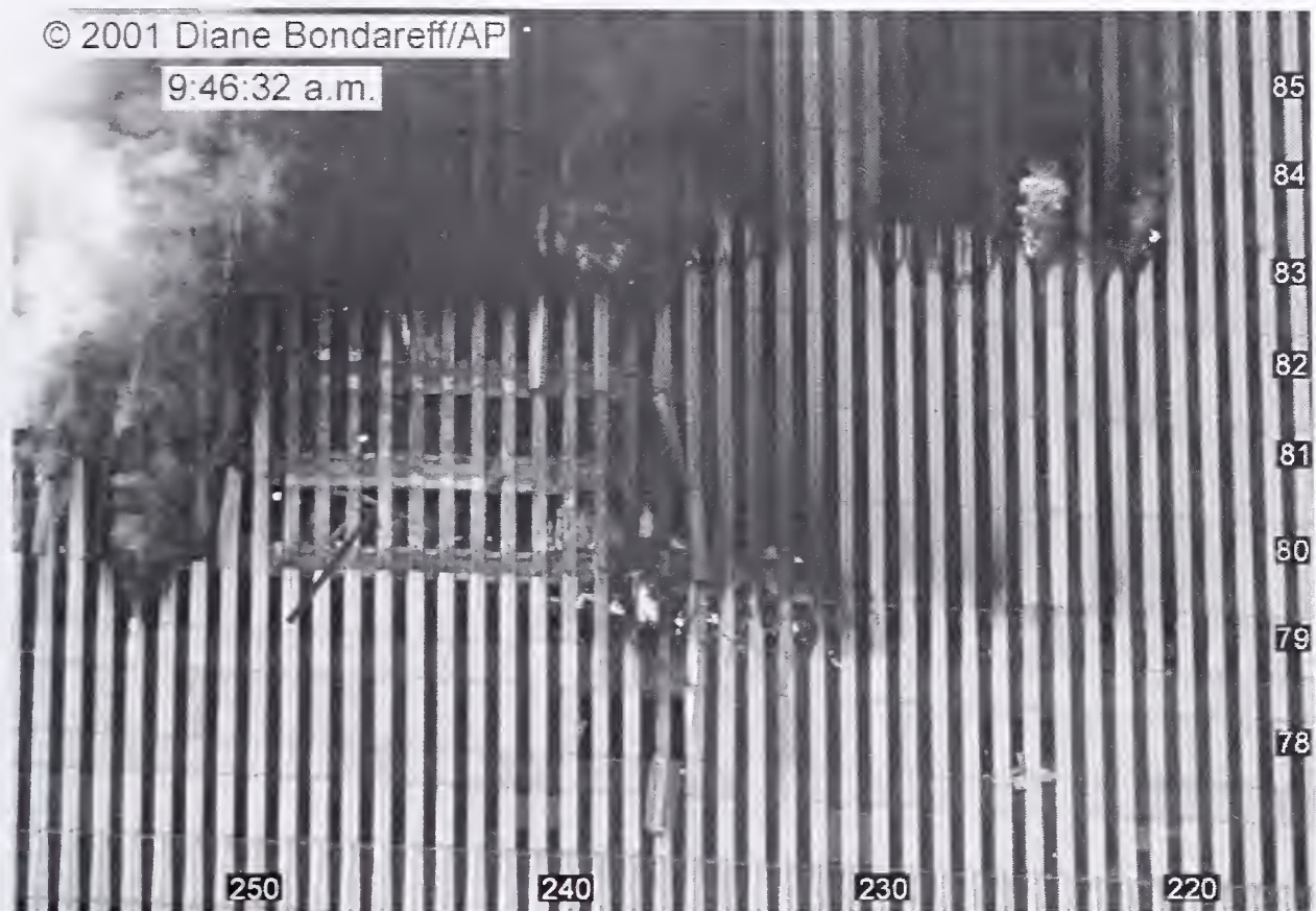
Figure 9-61. This cropped photograph shows the north face of WTC 1 at 9:46:32 a.m. The intensity levels have been adjusted, and column and floor numbers have been added. The arrow indicates a hanging object visible through windows on the 80th floor.
