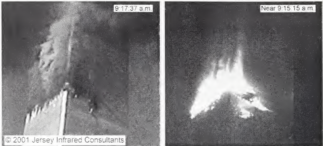
Figure 9-22. This figure compares an infrared photograph (on the right) and an image of WTC 2 captured from a video that was shot from the same vantage point and scaled and oriented to match the infrared shot. The north and east faces of the tower are visible. The video frame was shot at 9:17:37 a.m., and the infrared image was taken around 9:15:15 a.m. (an uncertainty of 15 s has been assigned).
