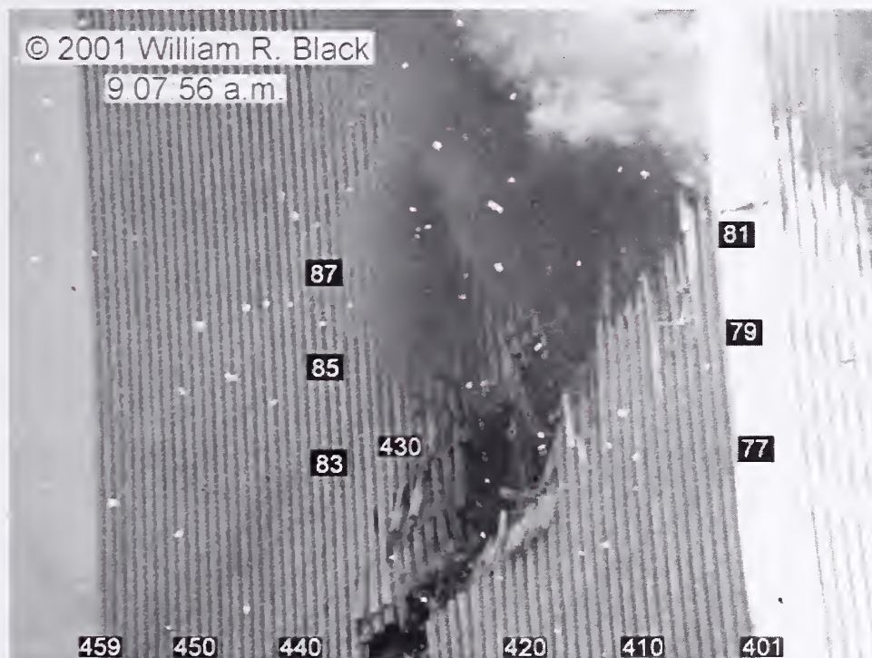
Figure 9-11. This photograph of WTC 2 was taken at 9:07:56 a.m. from the southeast and shows the south face and a portion of the east face. The intensity levels have been adjusted, and column and floor numbers have been added.
