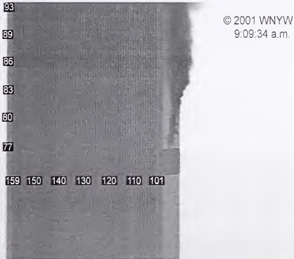
Figure 9-5. This image of the west face of WTC 2 was captured from a video shot from a news helicopter at 9:09:34 a.m. Column and floor numbers have been added.
