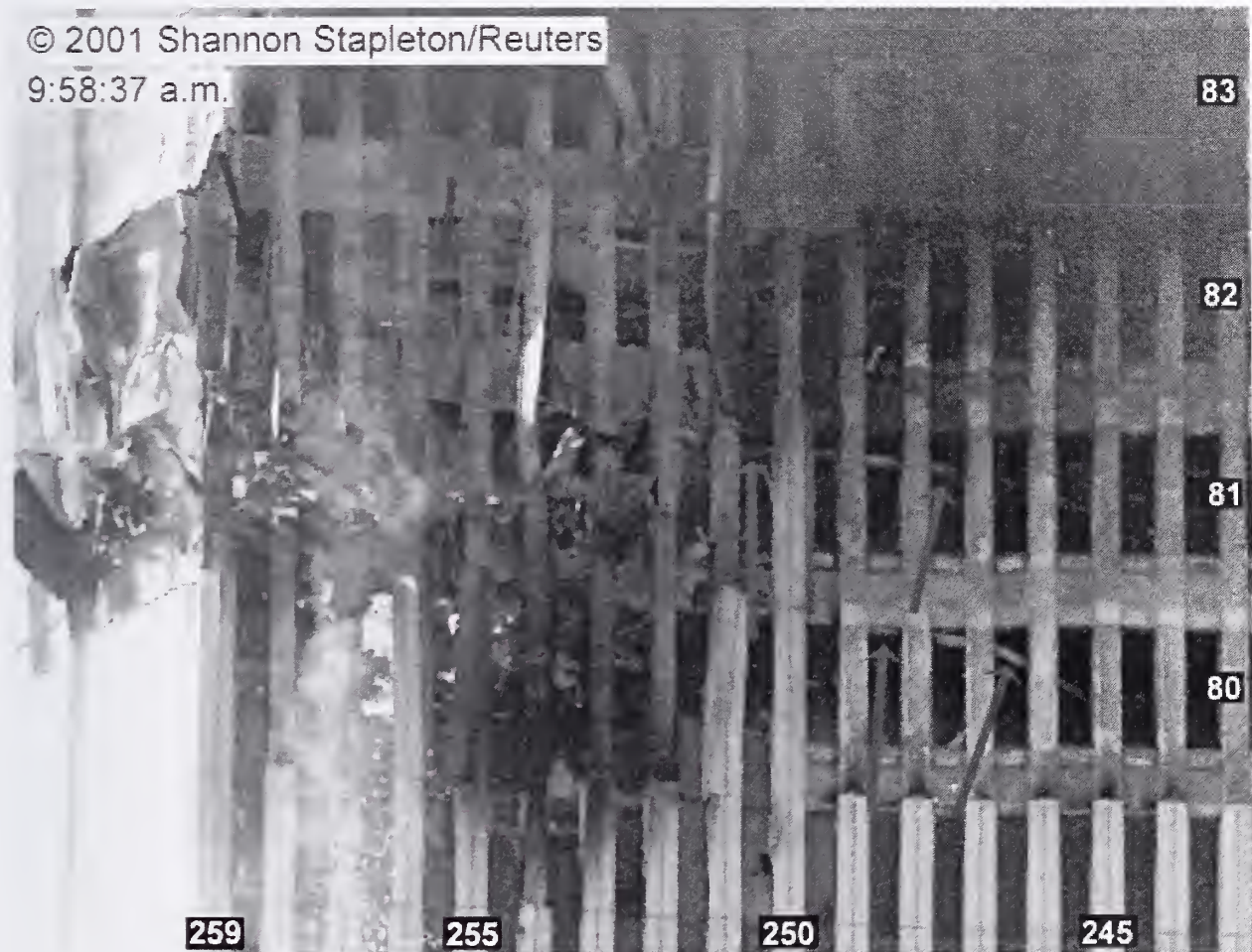
Figure 9-79. This photograph is a blow-up of a portion of the photograph shown in Figure 9-78. It shows the north face of WTC 2 and includes window 80-256 and part of the cold spot. The intensity levels of the original have been adjusted, and column and floor numbers have been added. Arrows highlight hanging objects visible through open windows on the 79th, 80th, 81st, and 82nd floors.
