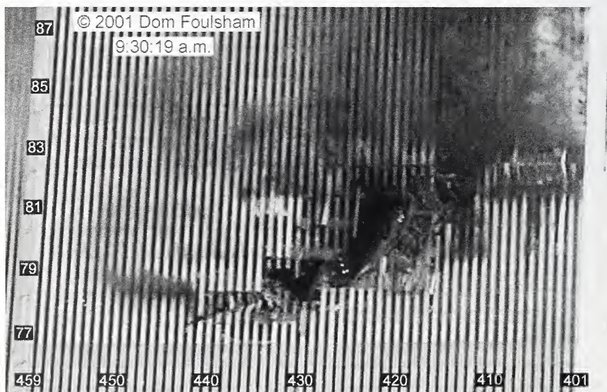
Figure 9-41. This cropped photograph shows the south face of WTC 2 at 9:30:19 a.m. The image has been rotated, and column and floor numbers have been added.
