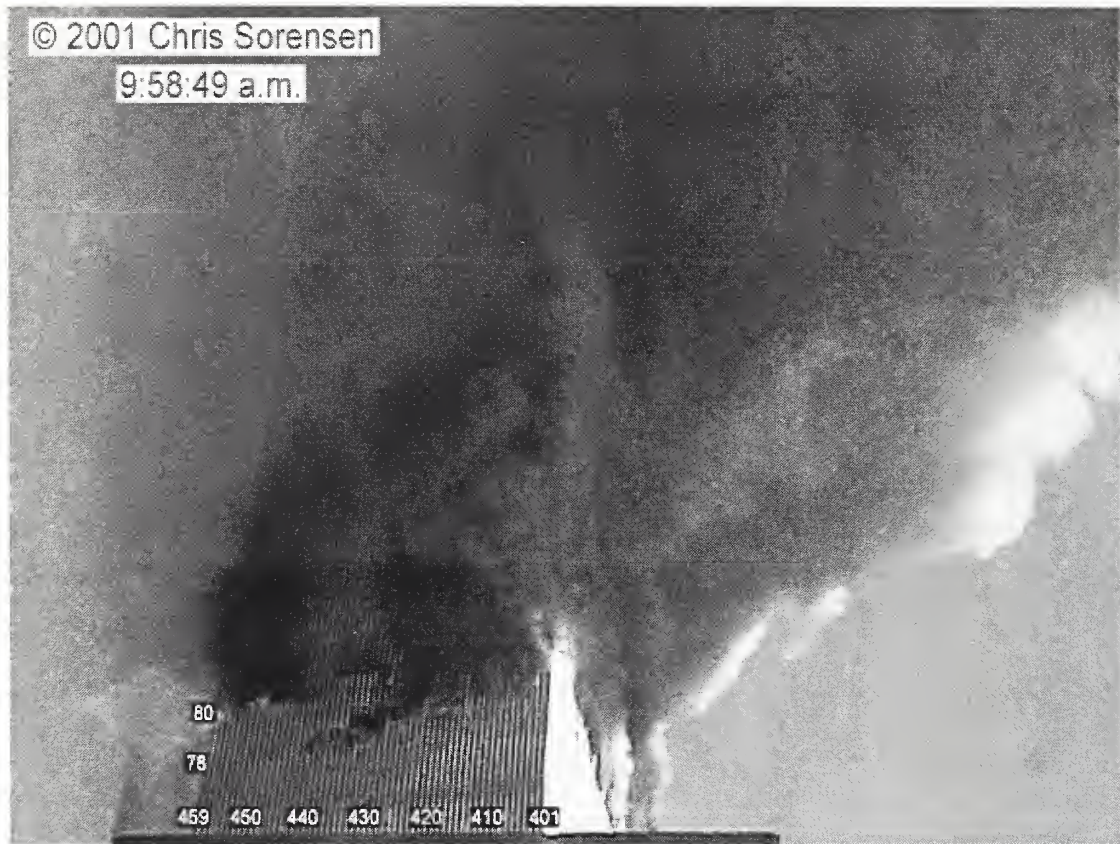
Figure 9-87. This image of the south face of WTC 2 is a frame captured from a video recorded at 9:58:49 a.m. The intensity levels have been adjusted, and column and floor numbers have been added.
