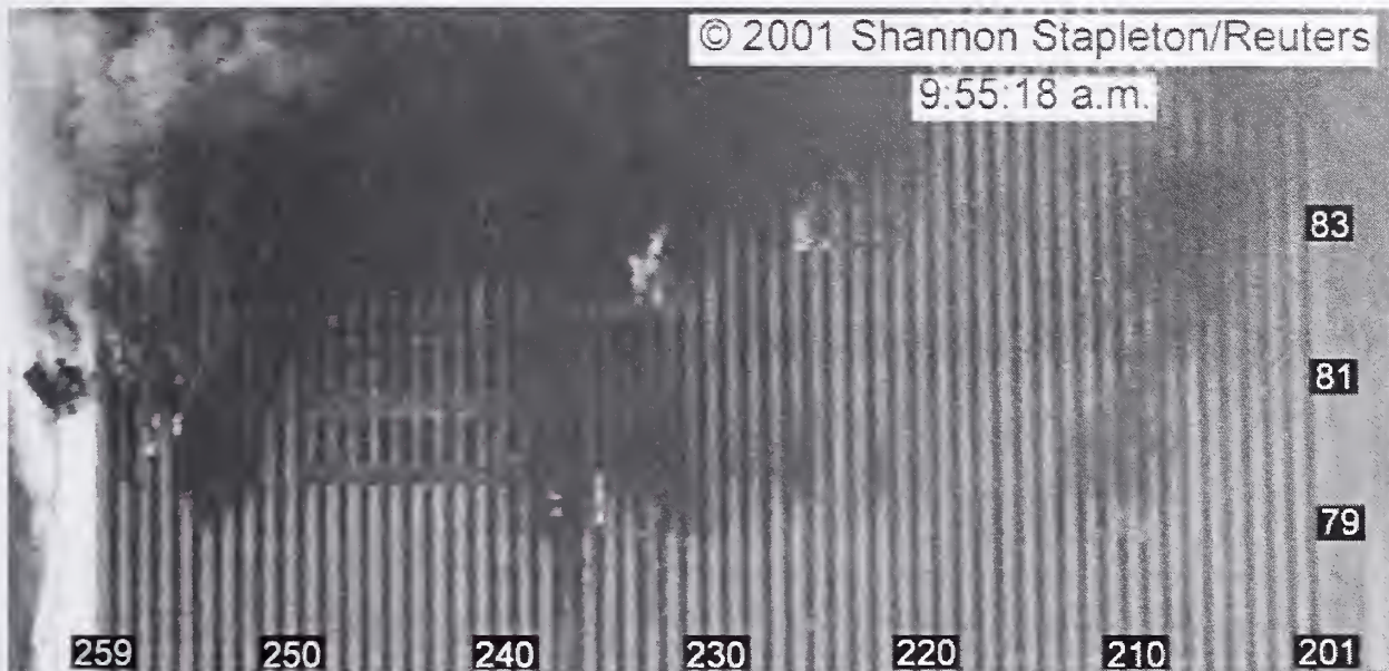
Figure 9-76. This cropped photograph shows the north face of WTC 2 at 9:55:18 a.m. The image has been rotated, and the intensity levels have been adjusted. Column and floor numbers have been added.
