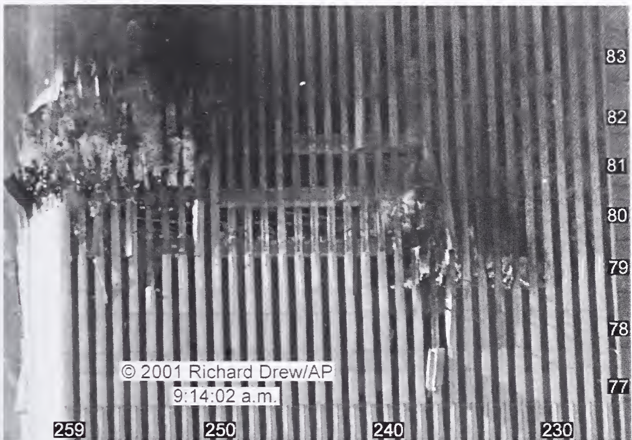
Figure 9-16. This close-up image of the north face of WTC 2 was taken at 9:14:02 a.m. The original photograph has been cropped and rotated, and the intensity levels have been adjusted. Column and floor numbers have been added. The arrows highlight hanging objects observed through open windows on the 80th and 81st floors. The brown area to the right is the eastern edge of WTC 7.
