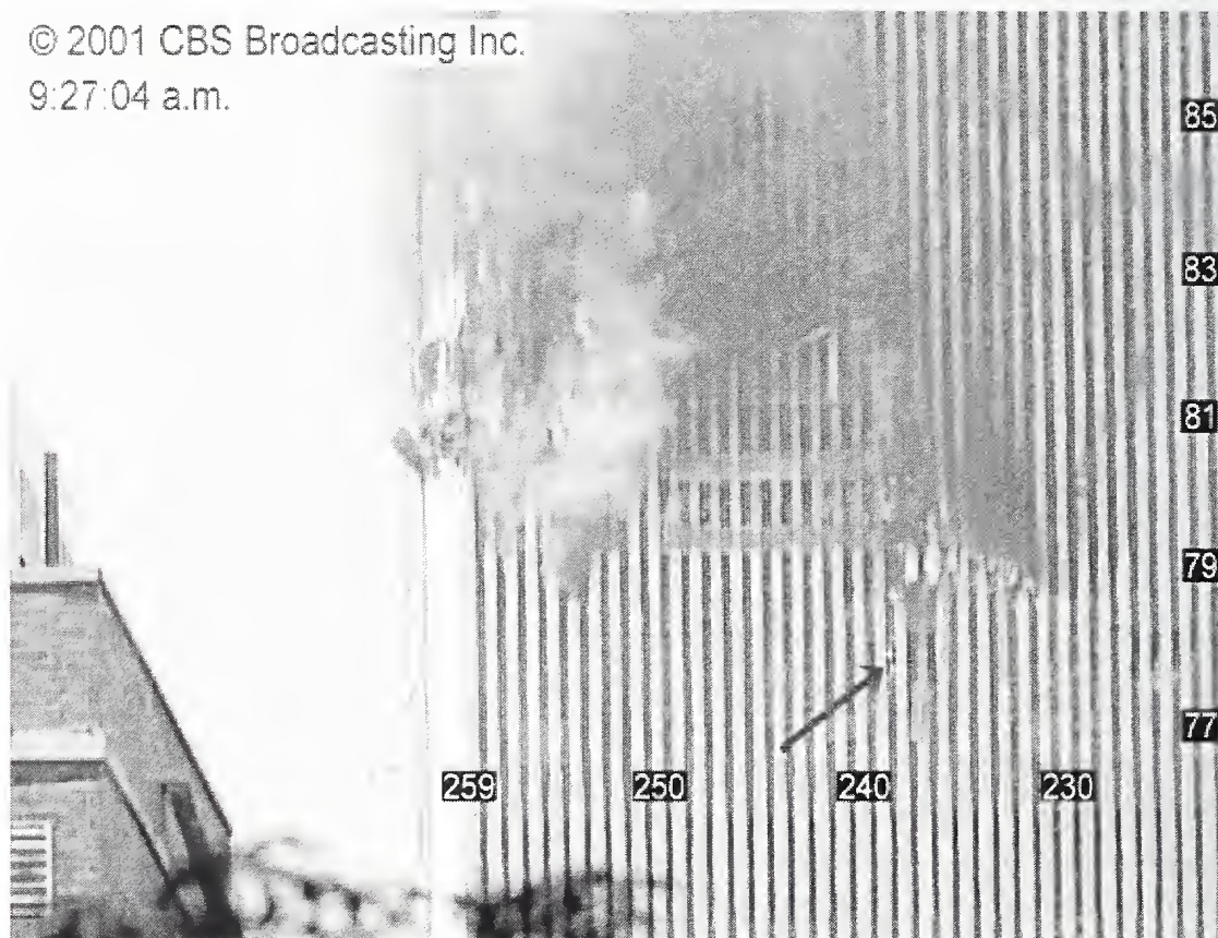
Figure 9-32. This captured video frame showing the north face of WTC 2 was recorded at 9:27:04 a.m. The intensity levels have been adjusted, and column and floor numbers have been added. The arrow indicates a stream of liquid-like material that was observed on the 78th floor falling in window 78-238.
