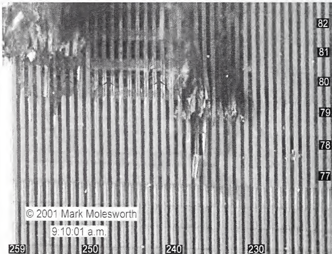
Figure 9-12. An image of the north face of WTC 2 captured from a video recording at 9:10:01 a.m. is shown. The intensity levels of the image have been adjusted, and column and floor numbers have been added. The arrows highlight hanging objects observed through open windows on the 80th floor.
