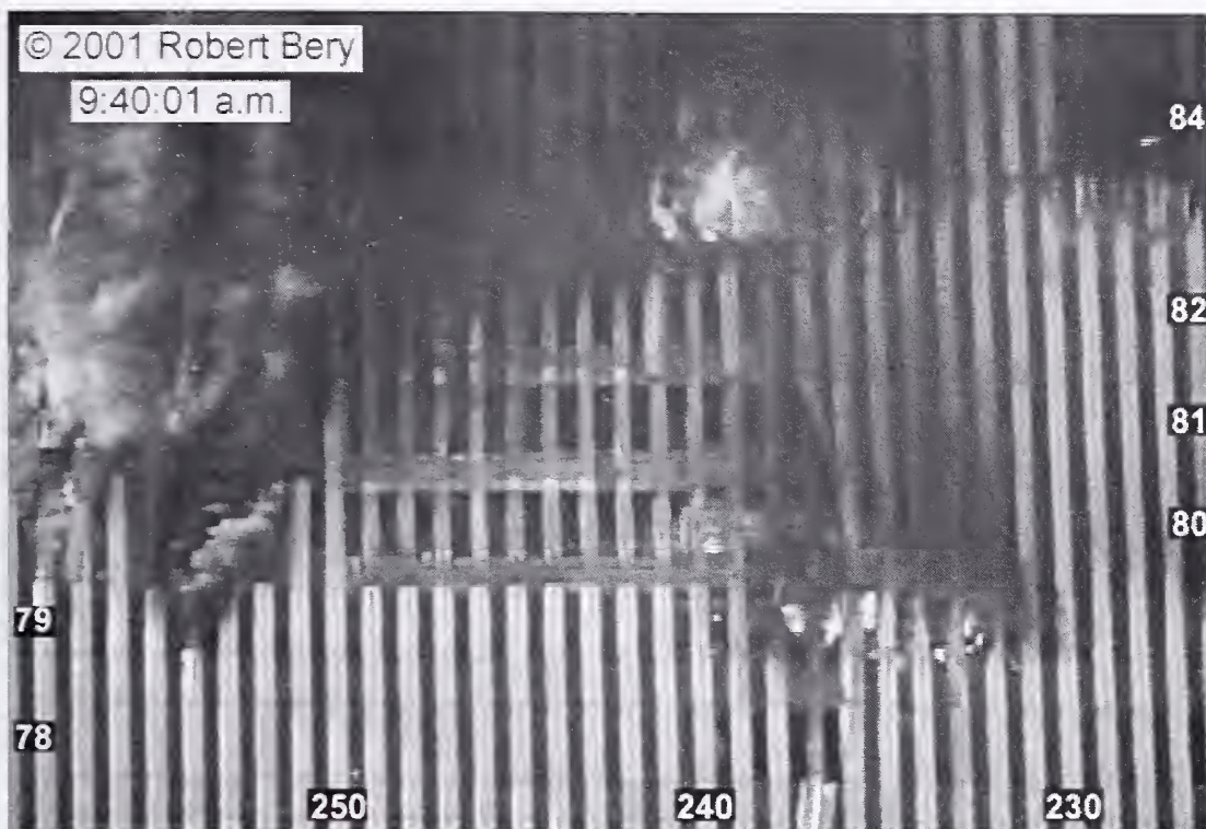
Figure 9-50. This frame captured from a video shows the north face of WTC 2 at 9:40:01 a.m. The intensity levels have been adjusted, and column and floor numbers have been added.
