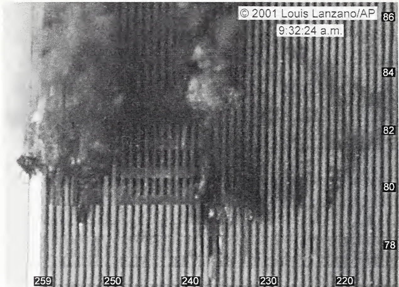
Figure 9-36. This cropped photograph shows the north face of WTC 2 at 9:32:24 a.m. The image has been rotated and enhanced by adjusting the intensities. Column and floor numbers have been added.
