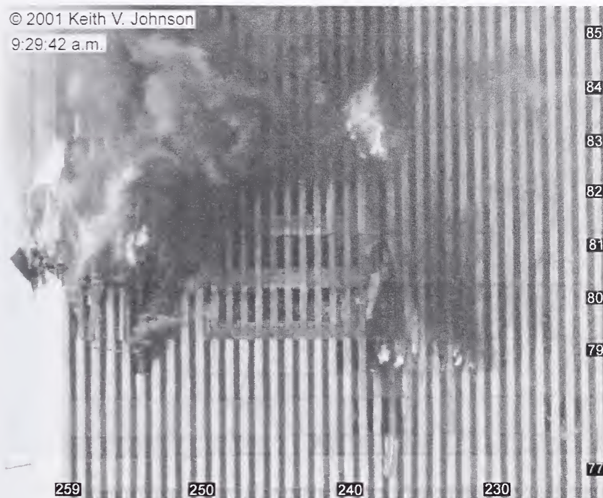
Figure 9-35. This cropped photograph shows the north face of WTC 2 at 9:29:42 a.m. The intensity levels have been adjusted, and column and floor numbers have been added
