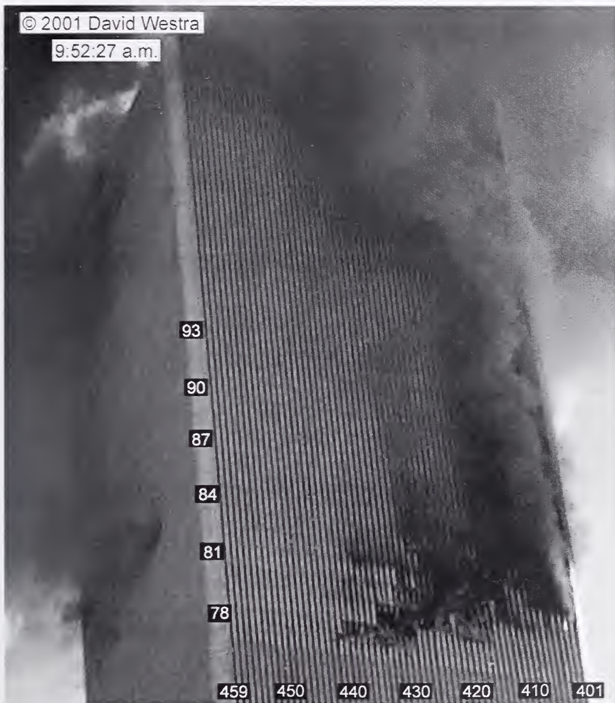
Figure 9-84. This cropped photograph shows the south and west faces of WTC 2 at 9:52:27 a.m. The intensity levels have been adjusted, and floor numbers have been added.
