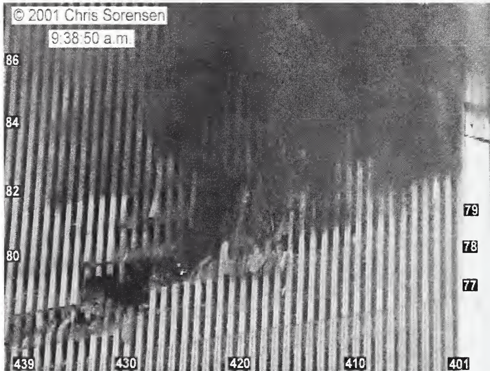
Figure 9-55. This image of the south face of WTC 2 was captured from a video recorded at 9:38:50 a.m. The intensity levels have been adjusted, and column and floor numbers have been added.
