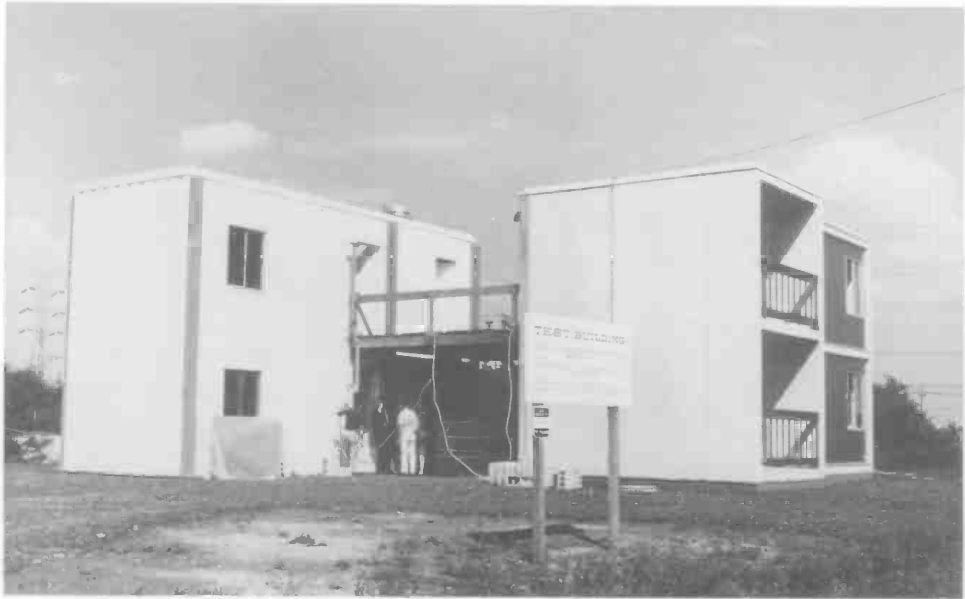
NBS engineers and technicians made last-minute inspections of the instrumentation used to monitor the full-scale burnout of the test building designed by the Pratt Institute. The steel wing (left) and the concrete wing (right) were joined by wooden stairs and a platform.
