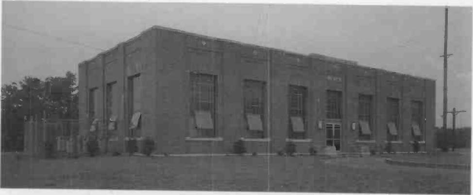
Exterior of NBS radio broadcasting station WWV, Greenbelt, Maryland. From this station, standard radio frequencies of 2.5, 5, 10, 15, 20, and 25 Mc were transmitted continuously. Two standard audio frequencies, 600 and 400 cycles, were broadcast as modulations on each radio frequency.
