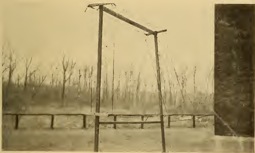
FIG. 30.—Coil aerial transmitter used at Navesink Lighthouse, 1916
