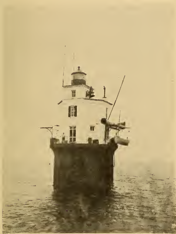
FIG. 35. Smith Point Lighthouse equipped experimentally as a radio beacon
