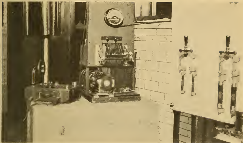
FIG. 29.—Early type of automatic radio beacon transmitter, installed at Navesink Lighthouse, 1916
