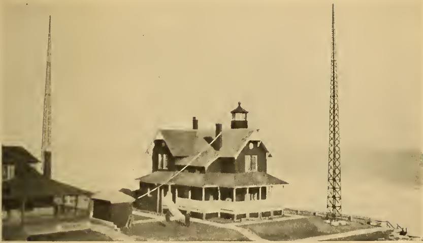
FIG. 36.— The Sea Girt Lighthouse equipped as a radio beacon
