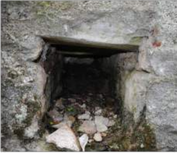
19. Opening for the removal of the discharges.
