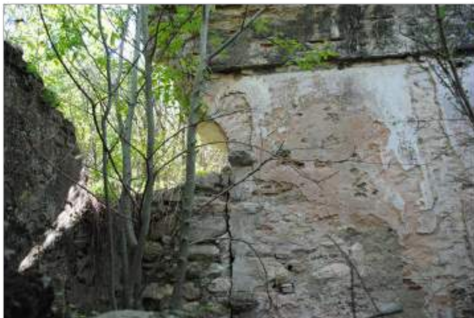
18. The locker room, view from the interior.
