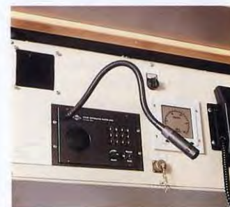
Amplidan command and talkback control station for internal communication
